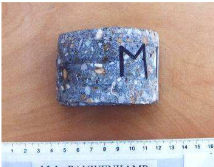
Figure: The need for further investigation: core drilling
