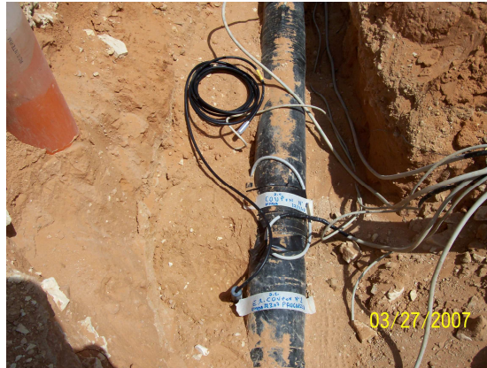
Installation of Coupon n. 1
