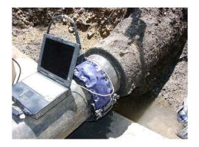
b – Flexible, pneumatically clamped system for larger diameter pipes
