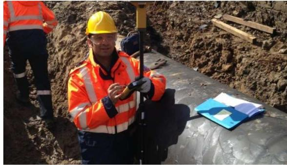
Figure 2, The survey pole shows the exact location of reported SCZ that was only 15cm away from the actual defect.
