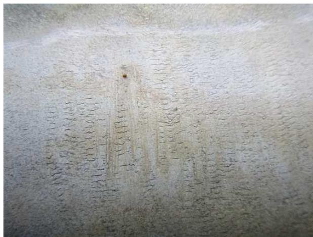
*Figure 4, Micro-cracks, with the longest one being 10mm.*
