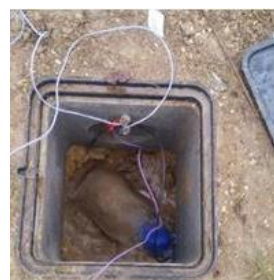
Figure 2 : RE model B (with bag) installation (just before backfilling)
