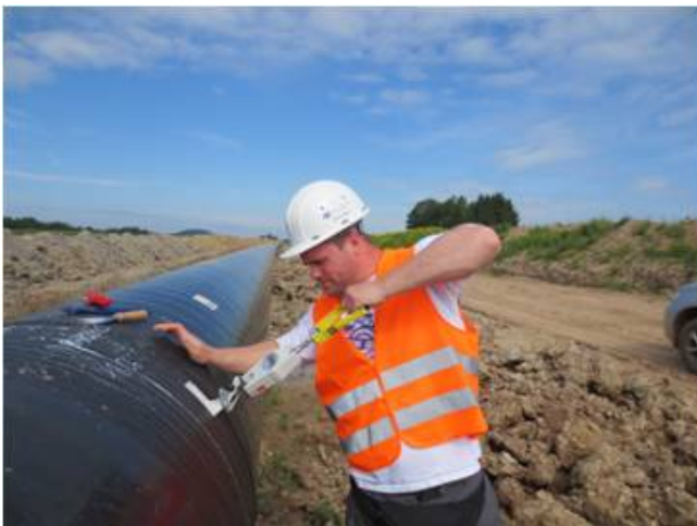
Figure 4: Destructive testing –peel resistance on cold applied PE/butyl rubber fjc
