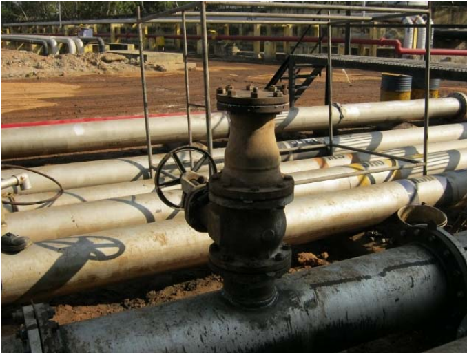
Fig. 3 – Short insertion spool
