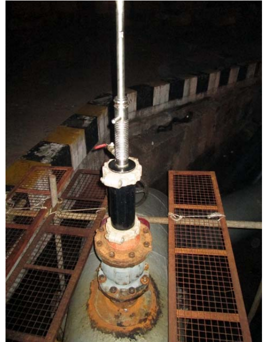
Fig. 4 – Hot-tapped insertion
