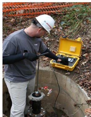
SmartBall ® insertion under live operating conditions
