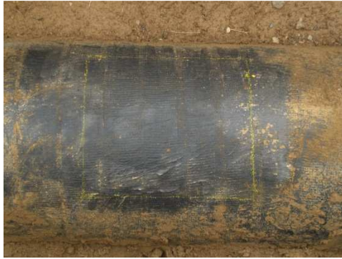
Fig. 4 Excavation – exposed ZMU
