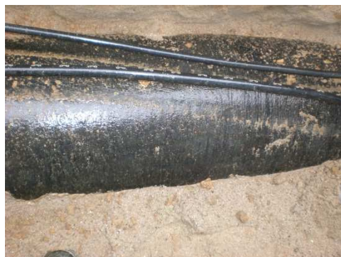
Fig. 6 Excavation – exposed ZMU
