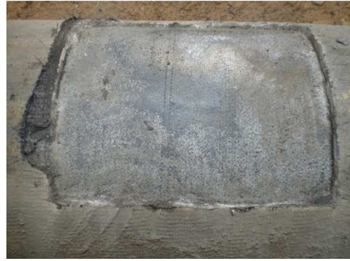
Fig. 5 Zinc coating with epoxy bonding layer
