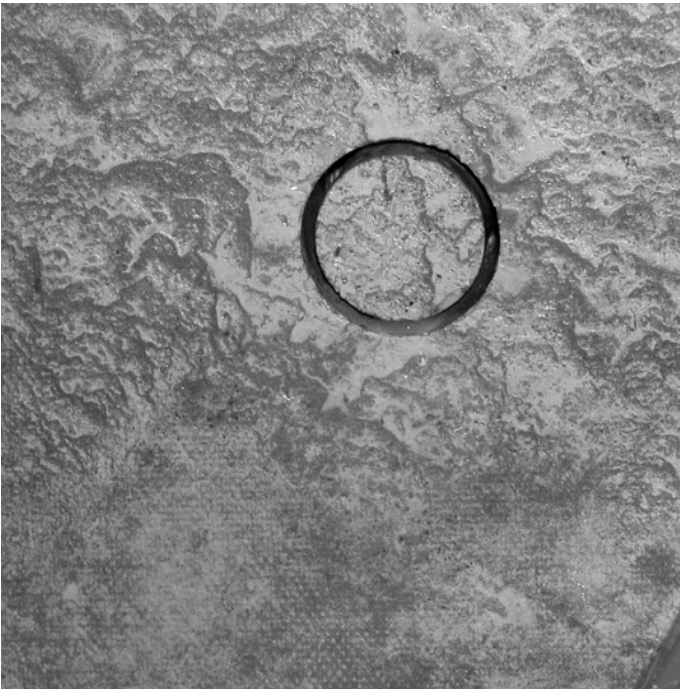
Fig. 13: Local cement slurry conservations
