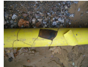
Figure 1: Pipeline constructed in the 1980s, coating made of PE [own photo]
