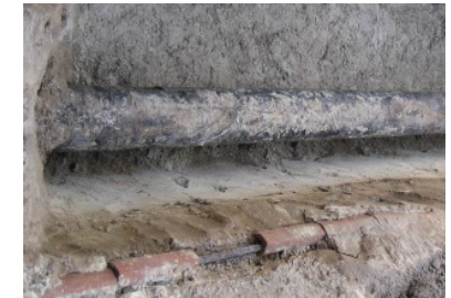
Figure 2: Pipeline constructed in 1954, coating made of bitumen [own photo]
