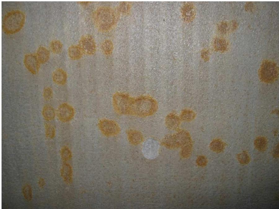
**Fig. 1: Formation of stains in a drinking water reservoir with mortar lining**
