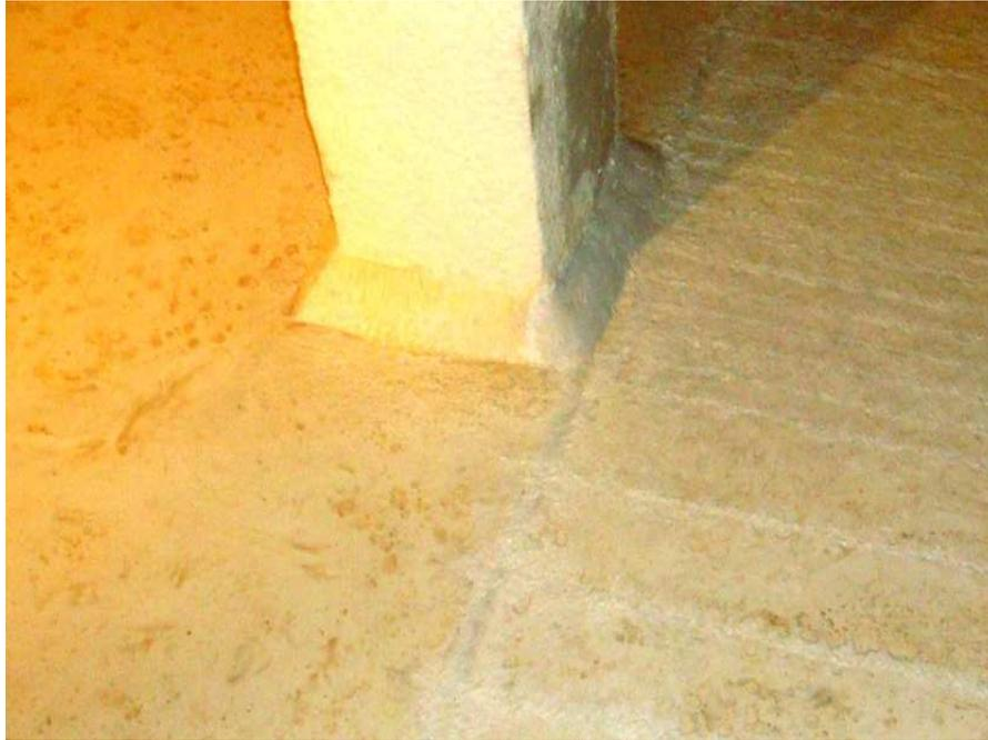
**Fig. 6:** Local formation of calcium carbonate at the concrete surface due to high protection current. Left side: no steel in concrete and no protection resulting in the formation of stains; right side steel wires embedded as cathodes in the concrete without formation of stains.
