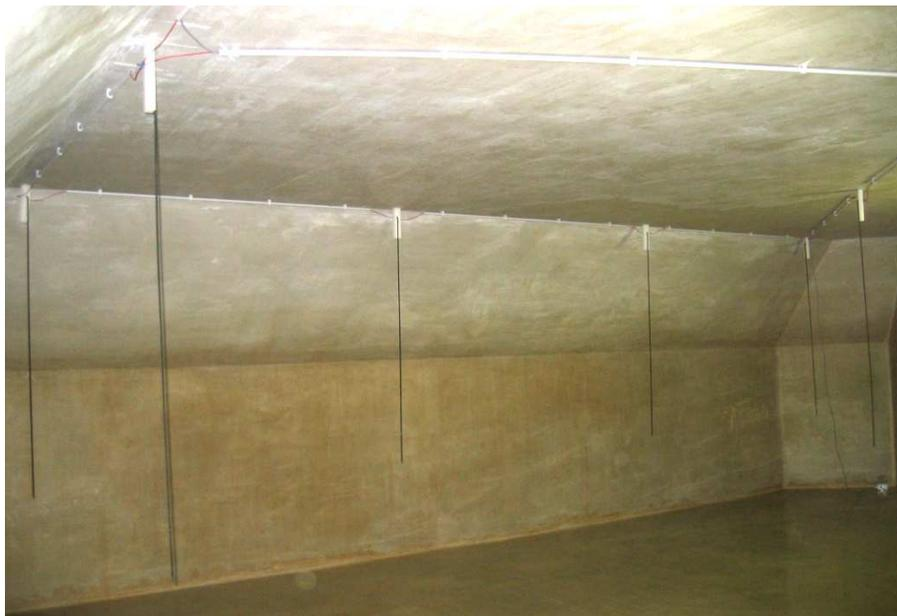
**Fig. 5:** Anodes installed in a water reservoir
