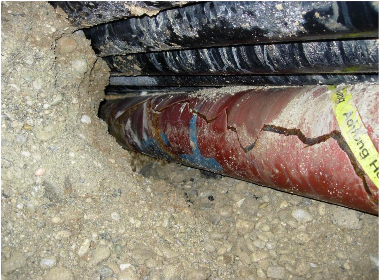
Figure 7: Desolate condition of pipe coating
