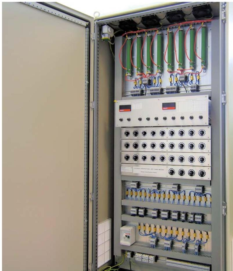
**Figure 5 – Traditional cabinet with resistors to distribute different currents to the groundbeds**
