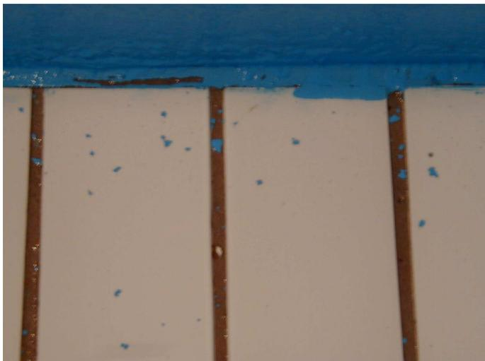
Figure 1: Flaking of a coating
