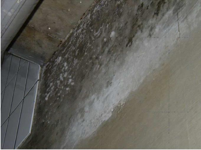
Figure 2: Fungus on a mortar surface
