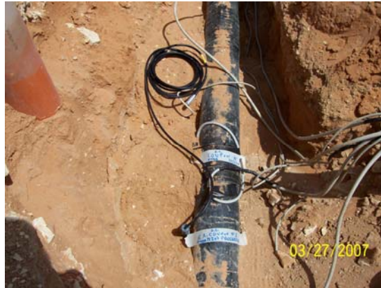
Installation of Coupon n. 1
