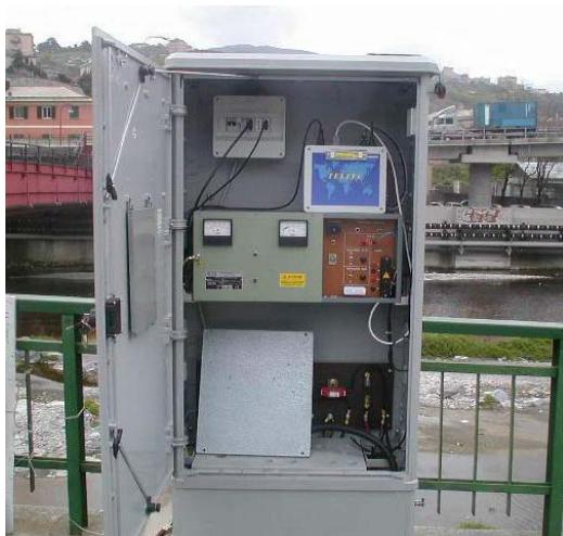
Picture 4: a test point with remote control unit on electro-mechanic power supply
