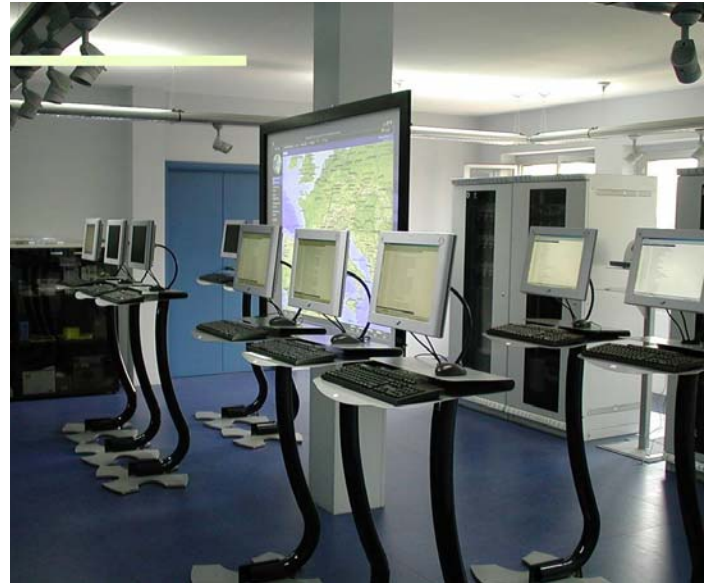
Picture 10: the Data Center
