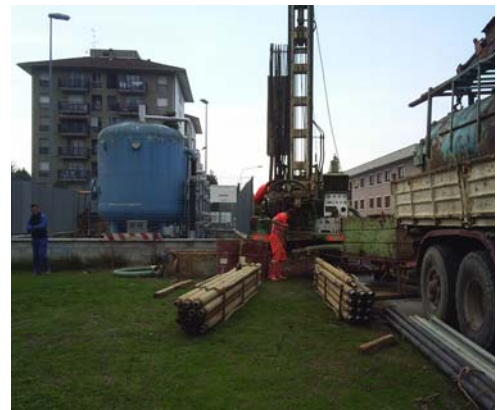
Picture 2: image of yard with drill
