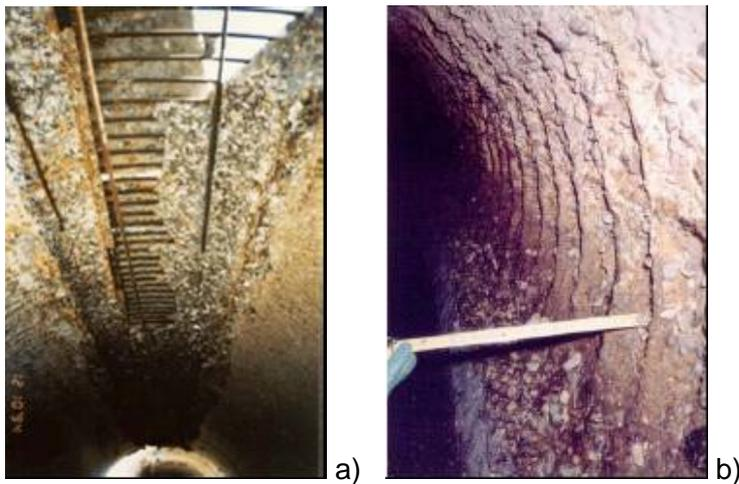
Figure 4: a) Corrosion by  $H_2SO_4$  of the crown composed of ordinary Portland concrete b) Uncovered reinforcements after less than 10 years of service of ordinary Portland cement pipes
