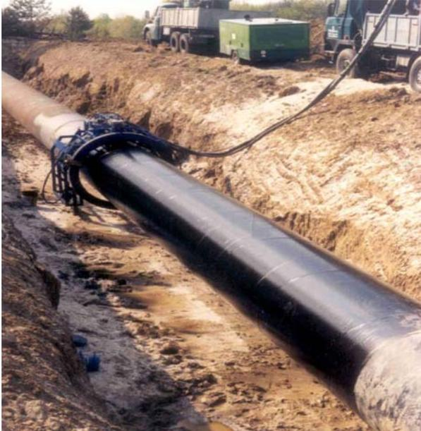
Figure 6: Belhole rehabilitation
