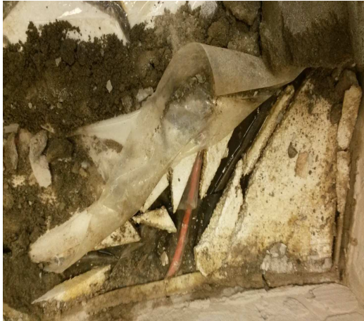
Figure 1: Water system installation between layers of waterproof material
