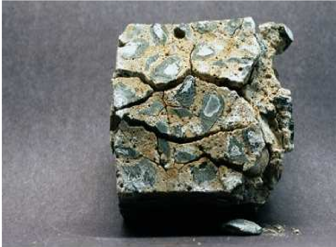
Figure 3: Biogenic sulfuric acid formation and the effects on a concrete cube.
